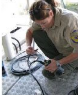
Connecting the responders to the junction
